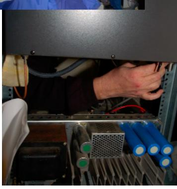
**BELOW** LEFT YOU **CAN SEE** THE **EXTERNAL POWER SUPPLY BELOW THE ICOM 440** REPEATER. LARRY HAS TO LAY ON FLOOR TO **ATTACH** THE WIRING.
