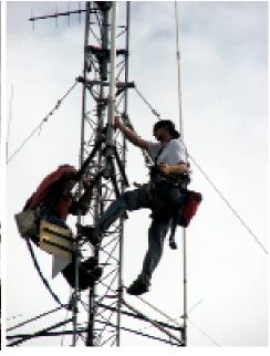
Work being done on Larry's tower, KA9KDC, this past Tuesday afternoon by Tower Works (a commercial tower company. This work was necessitated after tornado that plowed through Wheaton on the Afternoon of August 23rd. Left picture shows the clubs 2M antenna being realigned to the vertical position. Work also preformed by Tower included replacement of guy and structural hw. See the pictures in last month's Hamletter to note the differences.
