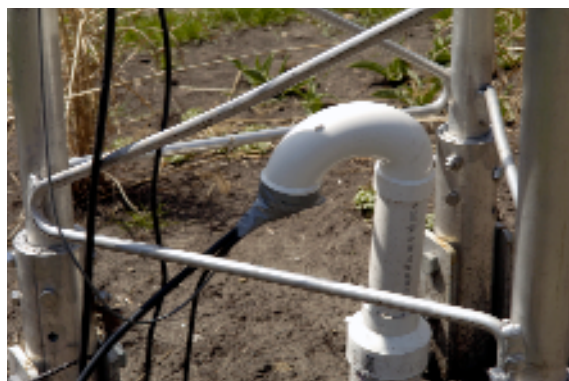
Coax feed into PVC for underground run to home entry point.
