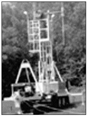
In this black and white photo, the antenna is assembled and the tower is on the way up.
